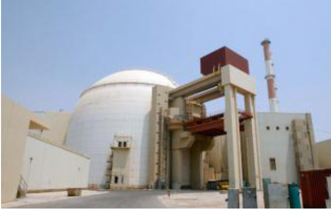
Figure 35: Bushehr power plant (Source: AP)
