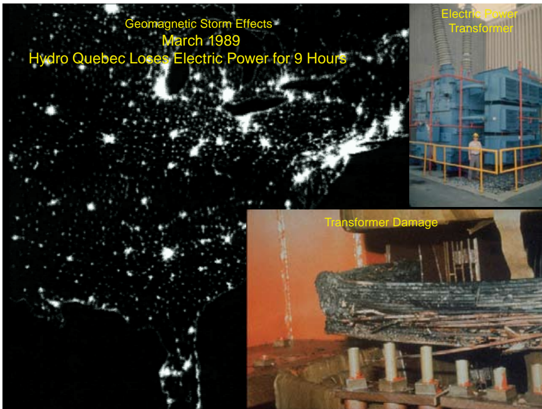
FIGURE 5.4 A 1989 geomagnetic storm caused a blackout in the Quebec region and damaged a high-voltage transformer. SOURCE: Rodney Viereck, NOAA Space Environment Center, “Space Weather: What Is It? How Will It Affect You?,” available at lasp.colorado.edu/~reu/summer-2007/presentations/SW_Intro_Viereck.ppt .
