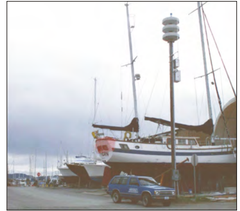
Figure 7. All Hazard Alert Broadcasting (AHAB) Radio on a pole installed October 30, 2003, Port of Port Townsend. Courtesy of the Washington Emergency Management Division.
