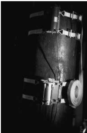
Figure 6 One of the pillars in the V2 building with an oscillating machine attached
